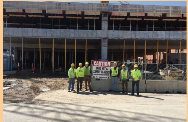
Local 140 Members at CD Smith Parking Ramp Project in La Crosse
