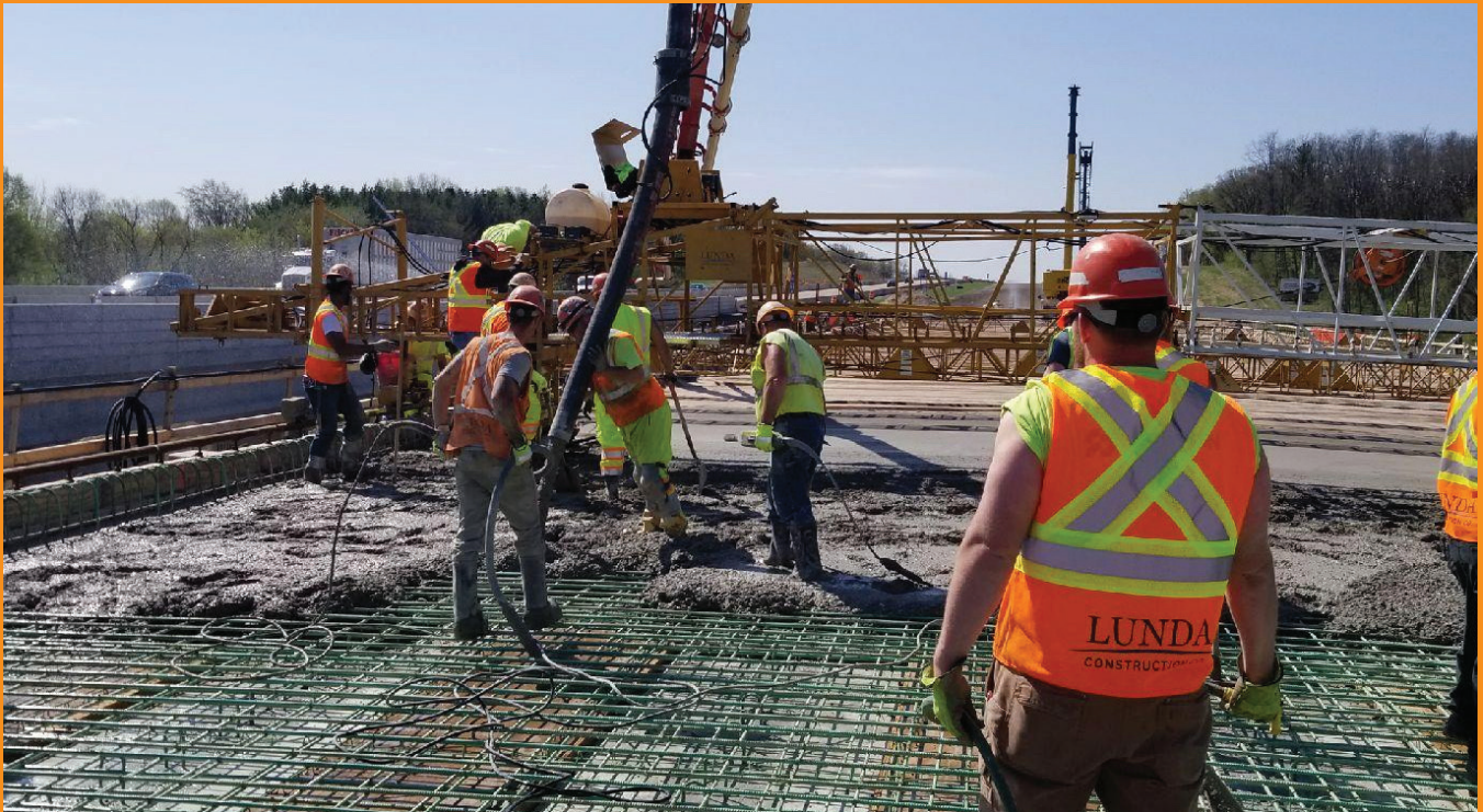
Members of Local 464 doing a concrete pour for Lunda Construction.
