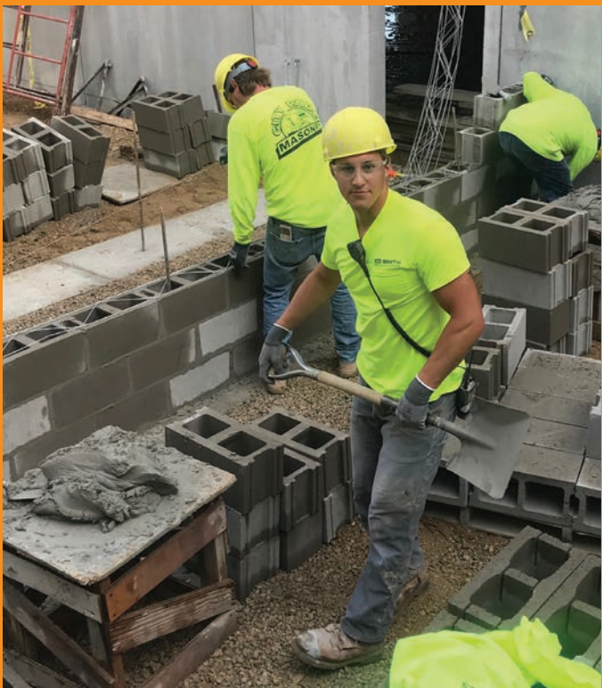
Local 113 Member Levi Kohn working on the Kewaskum School project.
