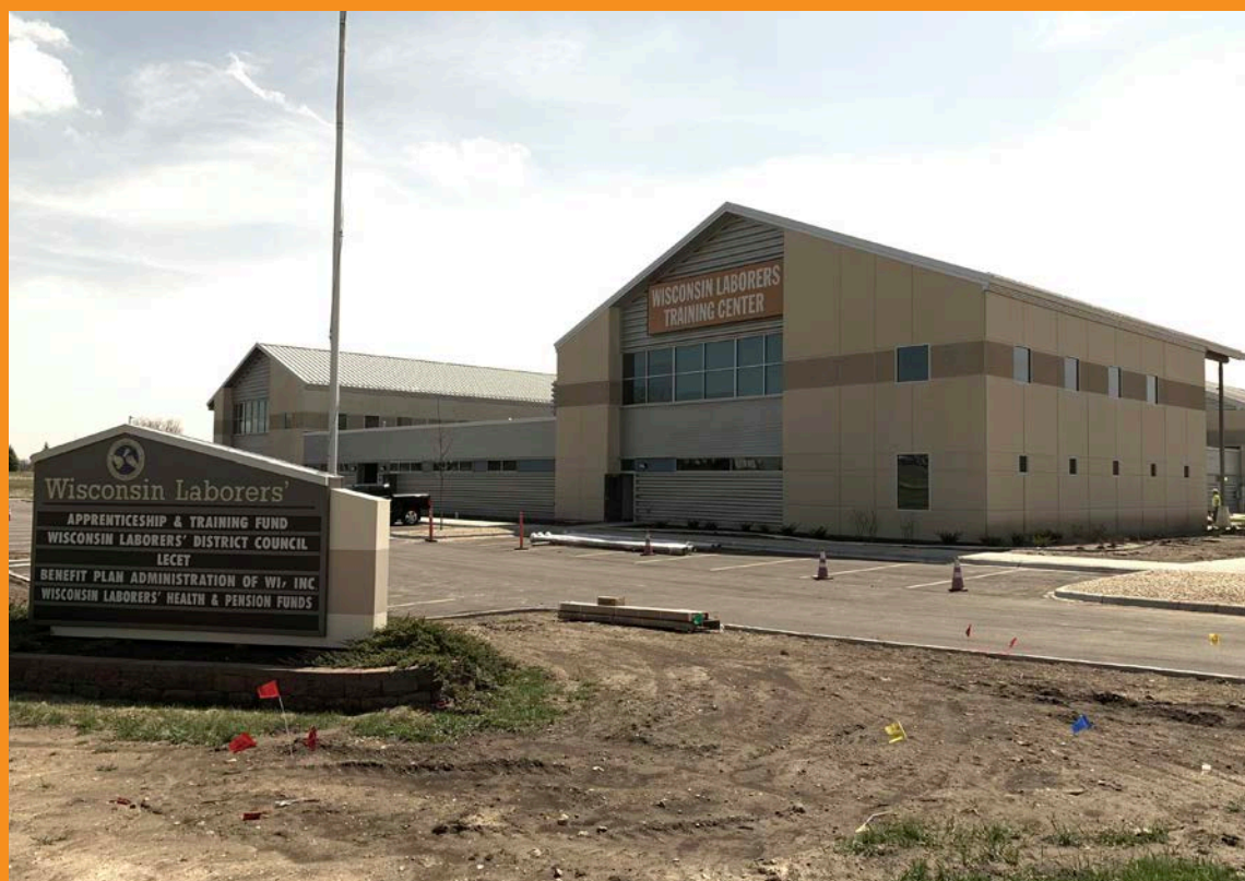
Above: The newly completed Training Center addition's environmental training bay and classrooms.
